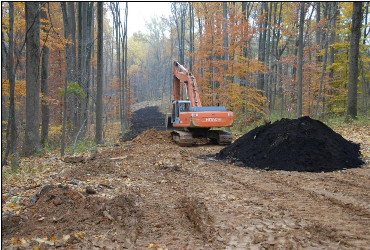
Excavator removing noncompaction layer and adding topsoil
