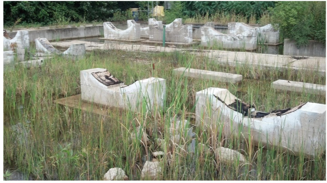
Former Tank Farm
