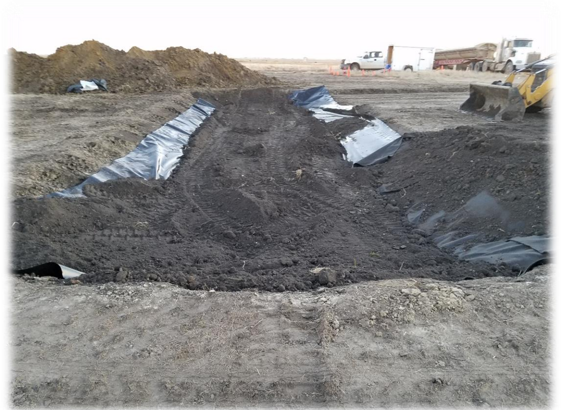
PRC-2 During Backfilling
