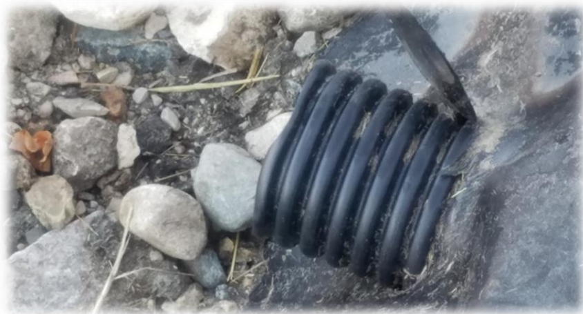
Drainage Outlet from Sump Pit
