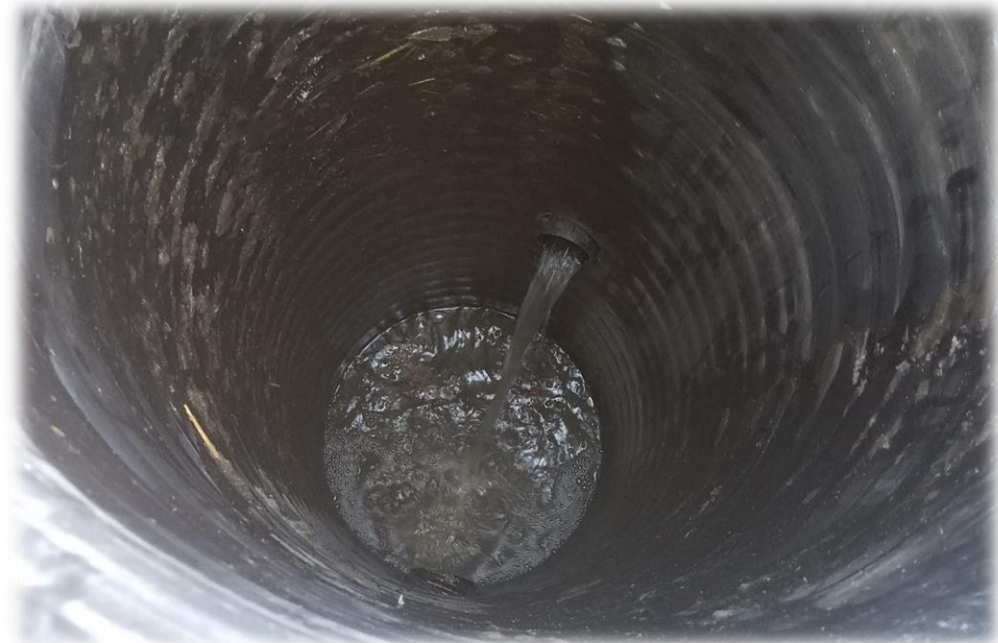
Water Draining from 3B into Catch Basin
