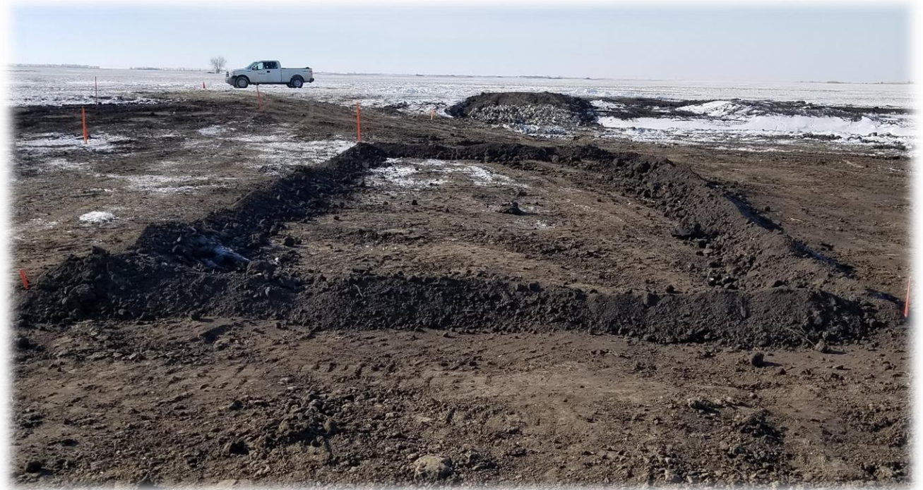
Test Plot 3A After Backfilling and Berm Construction
