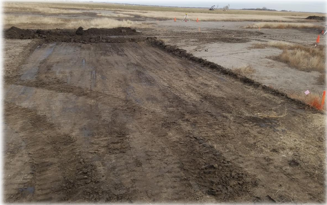
Test Plot 5B After 2-3% Grading
