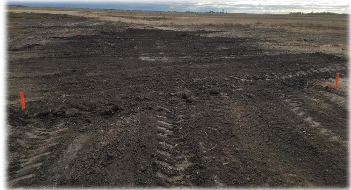
Test Plot 1A After Backfilling
