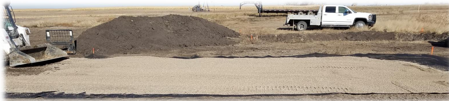
Placement of Geotextile and Pea Gravel as Capillary Break
