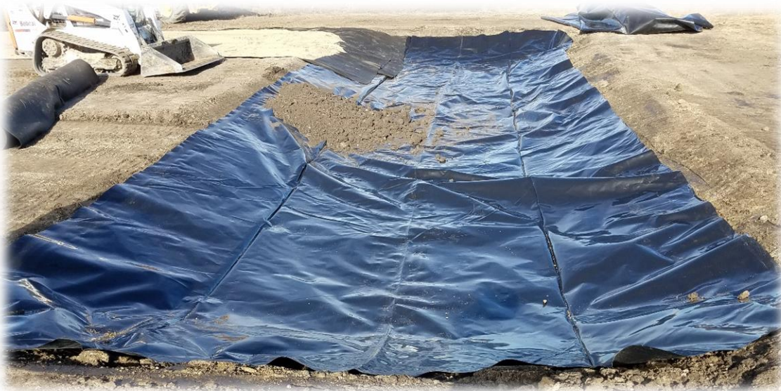
Impervious Liner Installed
