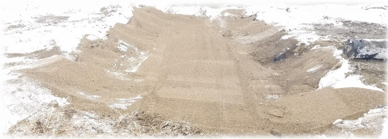
Drainage System and Pea Gravel Placed
