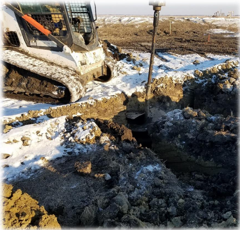
Sump Pit and Drainage Line Excavations
