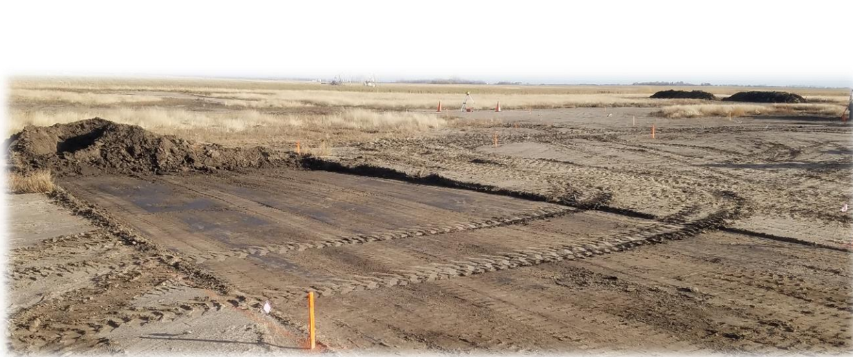
Test Plot 5A After 2-3% Grading
