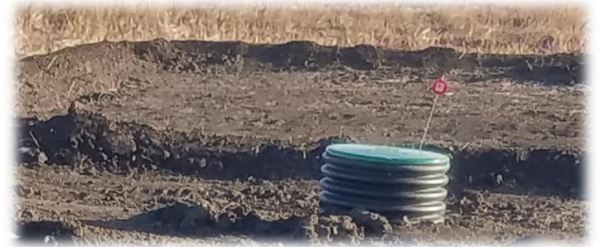
Catch Basin with Secured Lid and Reflective Marker
