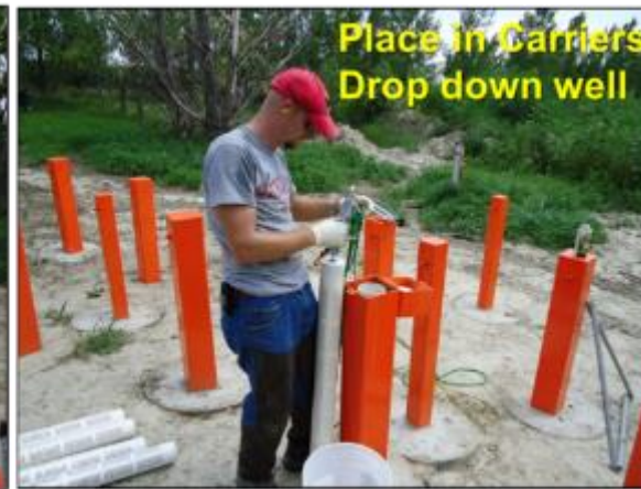
Added Aerators to Candles in Wells
