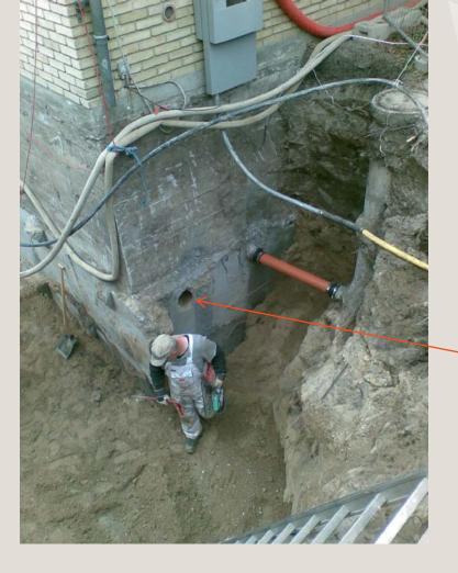
Hole from horizontal drilling
