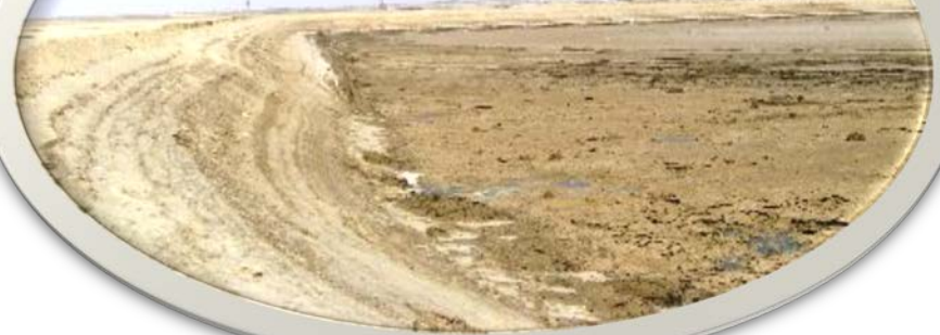
Effluent Pit C1- Before
