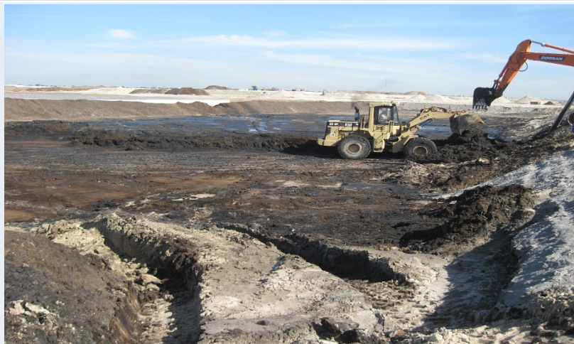
Wet Sludge Removal-1
