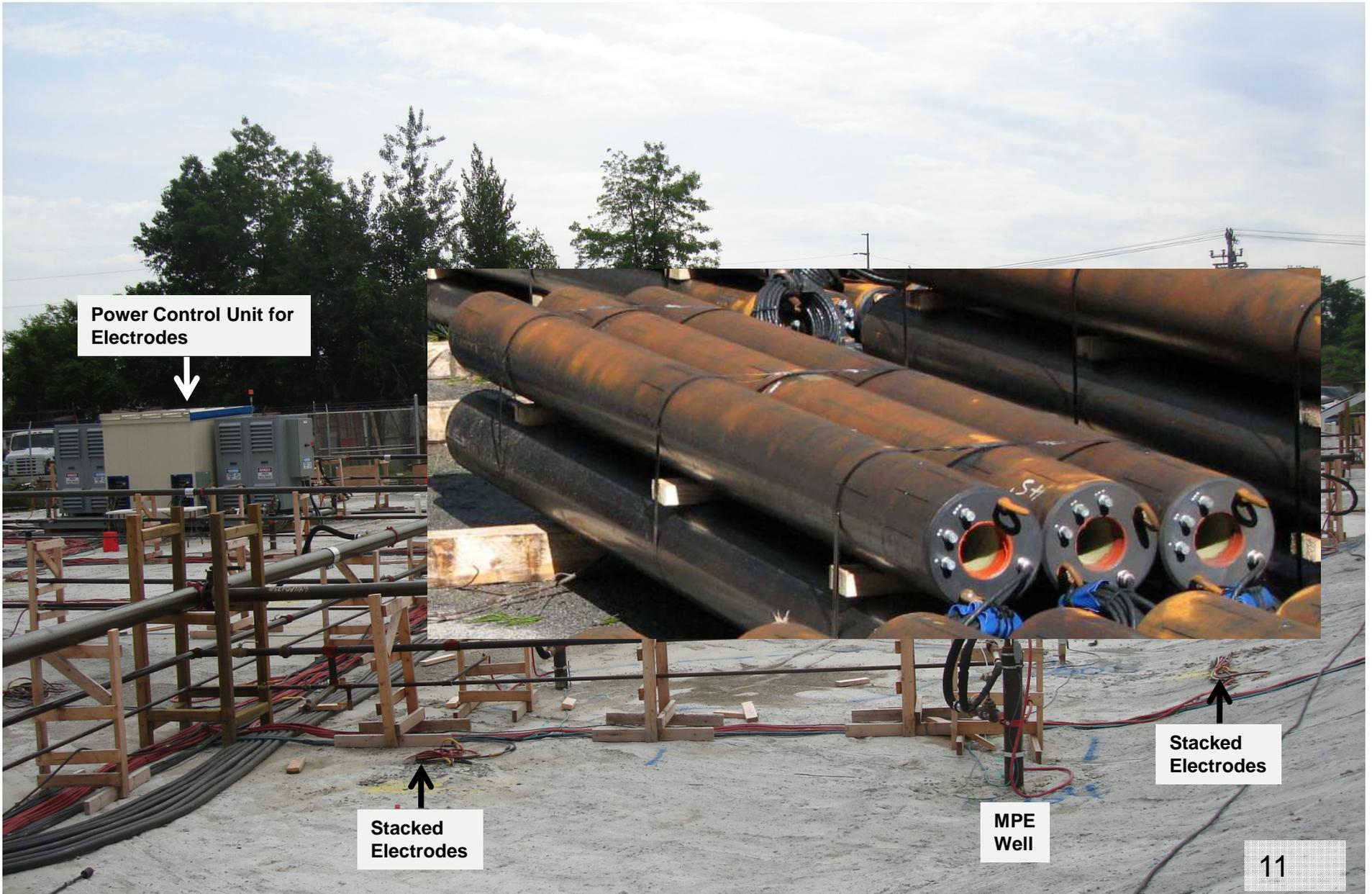
Power Control Unit for Electrodes
