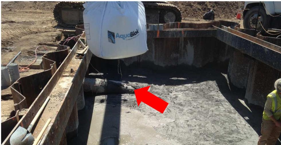
**Setting / Purpose:** Pipeline cap and Anti-Seep Collar. Objective was to cut off site contaminant pathways during excavation and installation of natural gas pipeline.
