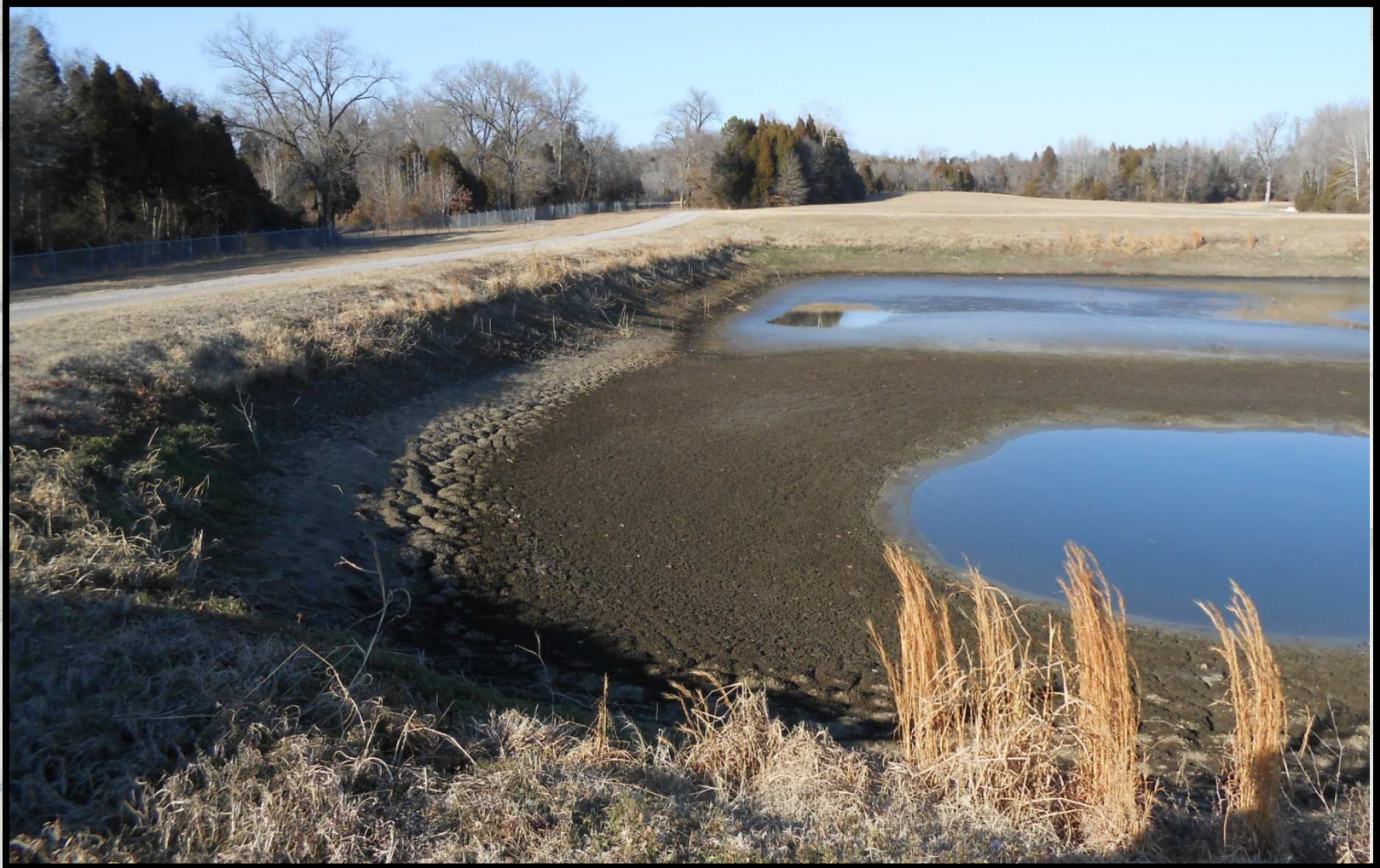
Fort Smith, AR – Water Treatment Detention Basin
