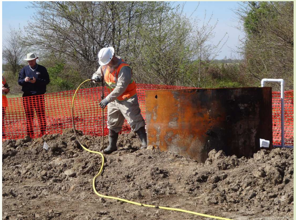
Cool-Ox ® Brine-Buster ™ Injection Application with DTI's Hydro-Dart ™ near the sump tank
