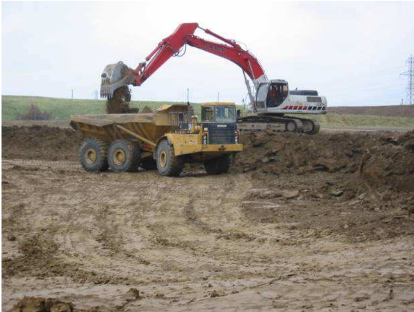
Excavation of Treatment Materials
