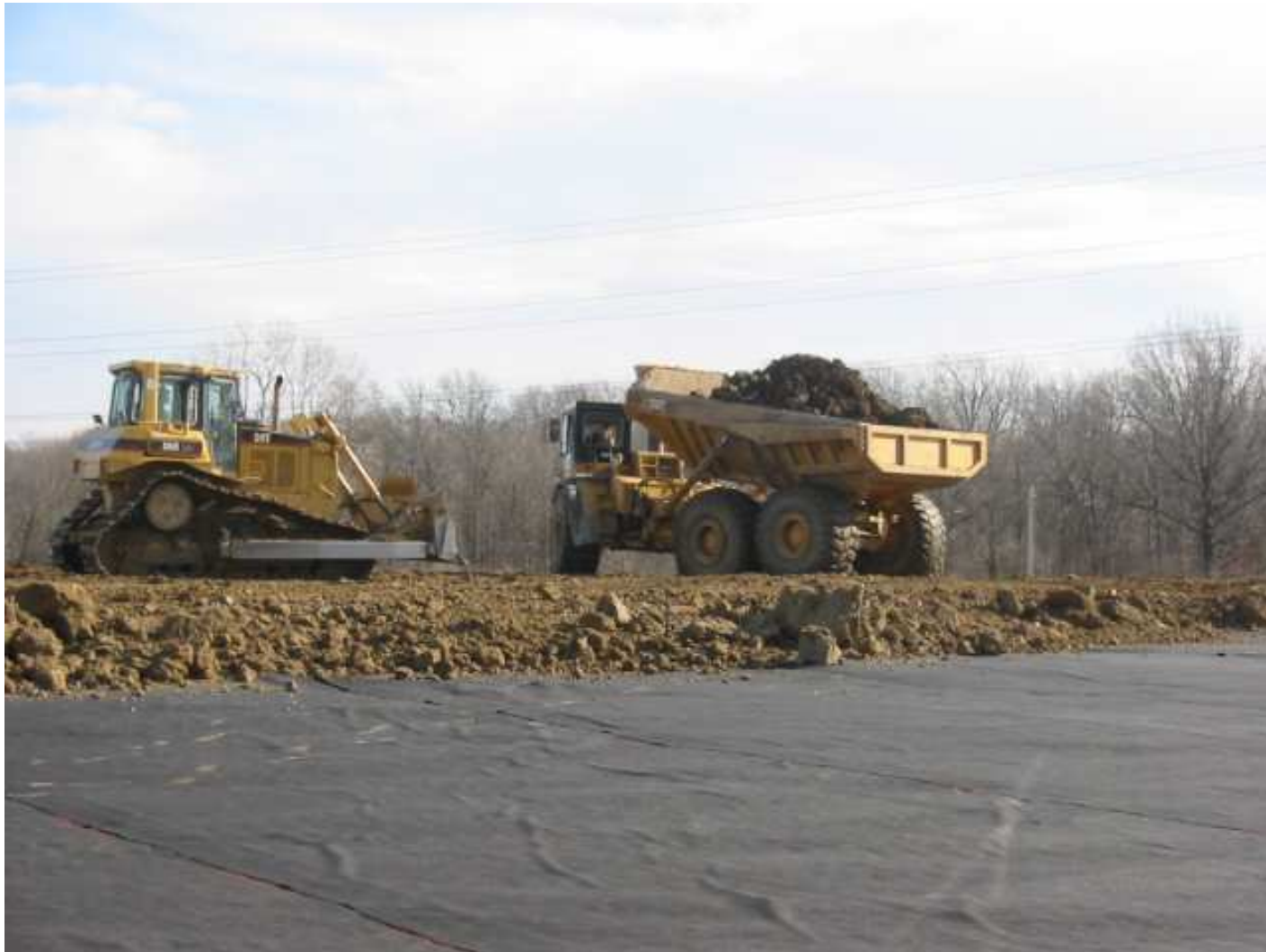
Placement of Soil Cover
