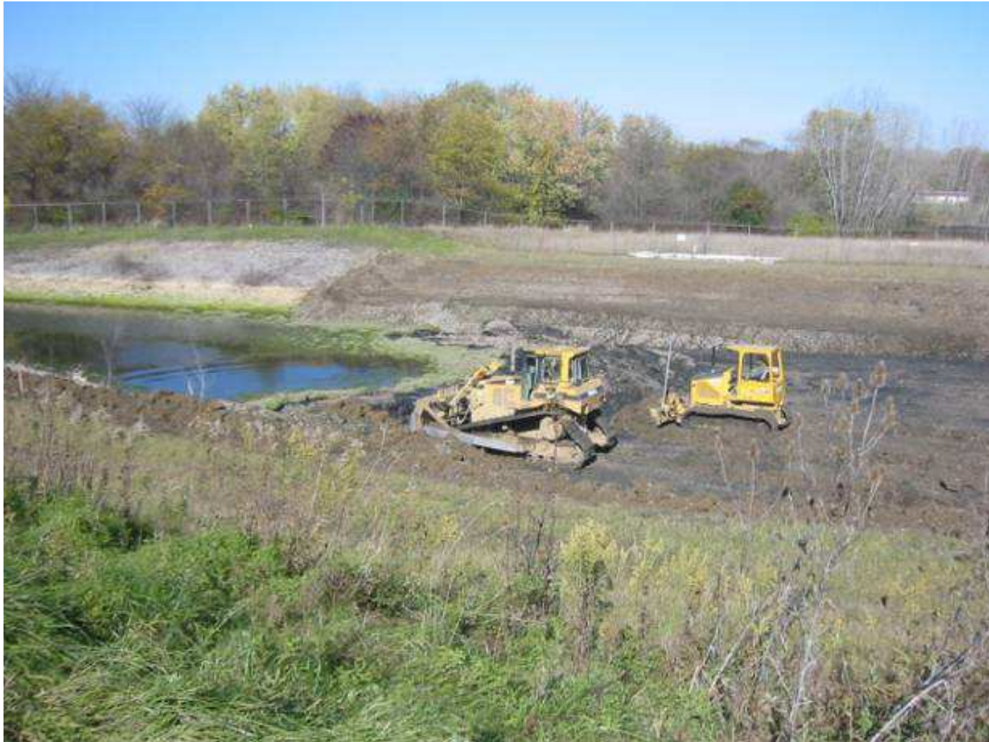
Excavation of Stormwater Pond Sediment
