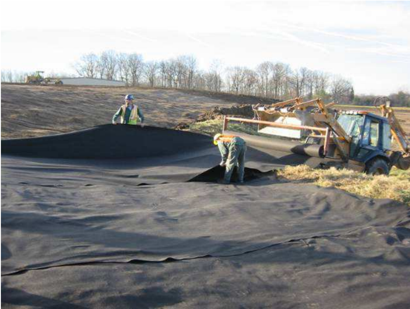
Installation of Root Penetration Barrier
