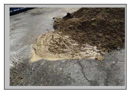
The contrast between treated contaminated soil (light tan color) and the backfill material.
