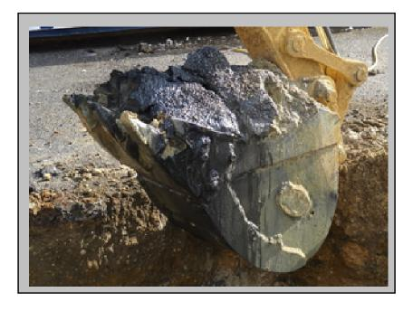
Although only mild soil contamination was referred to in the site data, free product was encountered once the soil/groundwater interface had been reached.
