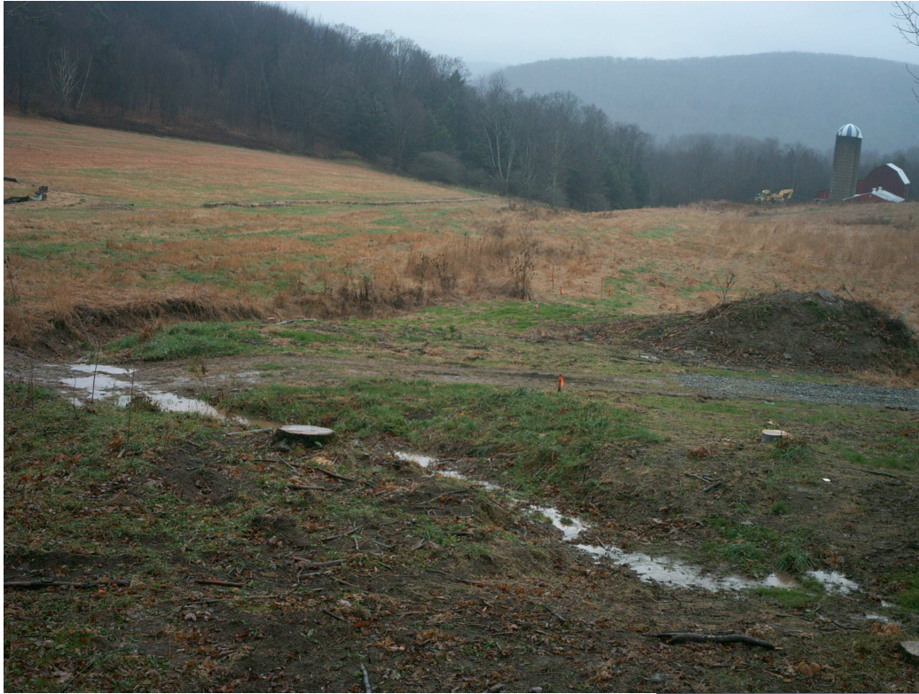
Degraded Stream Before Restoration
