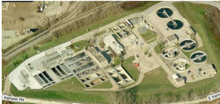
Bird’s eye view of a wastewater plant
