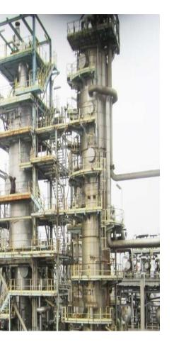
• FCCU takes higher molecular hydrocarbon and "cracks" them into more valuable lighter hydrocarbon compounds for gas and diesel
