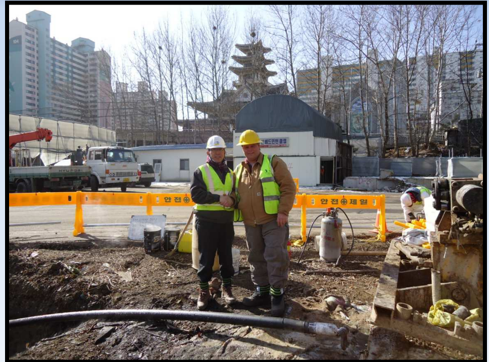
Installing first ever horizontal remediation wells (HRWs) in South Korea
