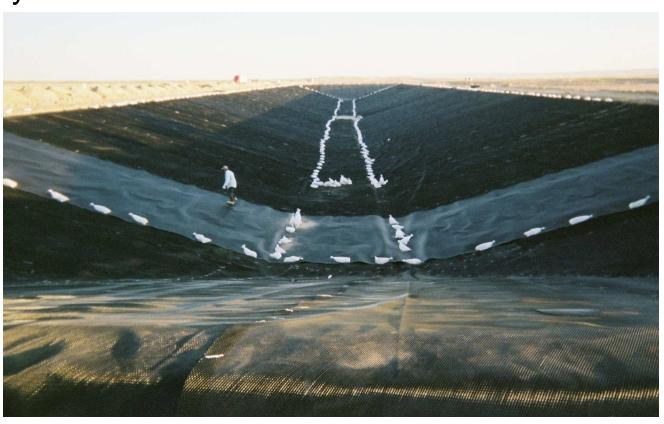
Ponds designed and constructed with two geomembranes over compacted clay or geosynthetic clay liner and a geonet and flat pipe leak layer in between to monitor the primary liner for leaks.
