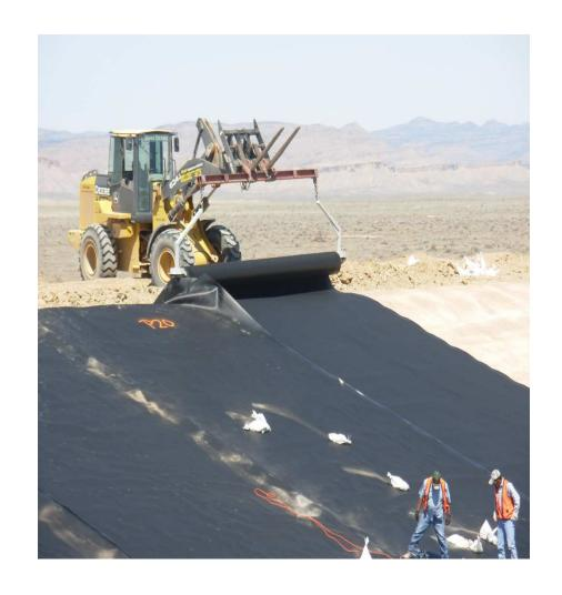
Geomembrane panels are welded together throughout the installation performed by trained and certified technicians.
