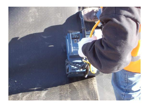
Geomembrane panels are tested for strength throughout the installation performed by trained and certified technicians.
