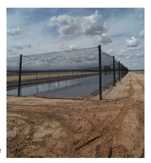
The water is fed by gravity or force main pipe to the evaporation ponds from the settlement/sludge pond or directly from the oil/water separation equipment.
