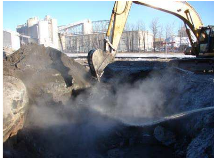
Excavating Look at the Bucket
